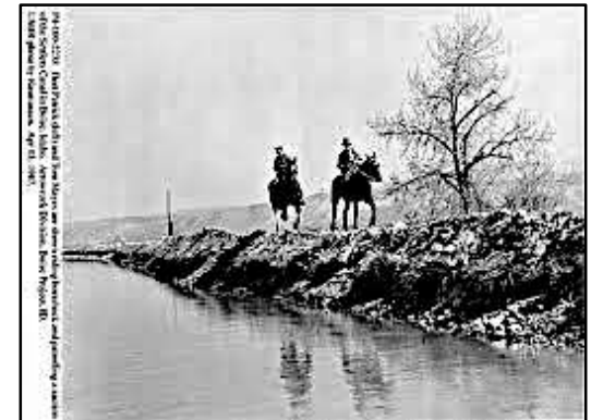
Ditchriders patrolling a section of the Settlers Canal in Boise, Idaho. Arrowrock Division, Boise Project, ID. USBR photo by Rasmussen. Apr 15, 1947
